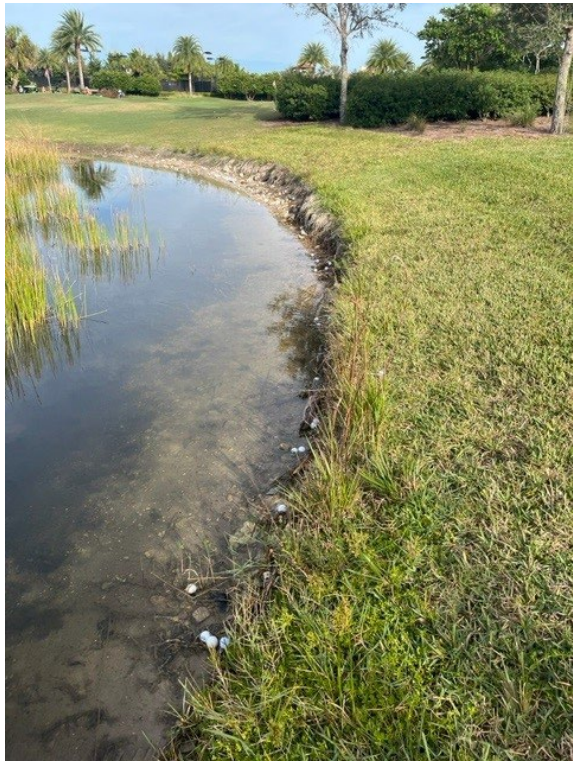
SWM - Lake Bank Slope (Aqua Range)
