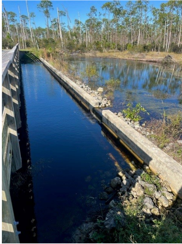
SWM - Flow Way Weir (North)
